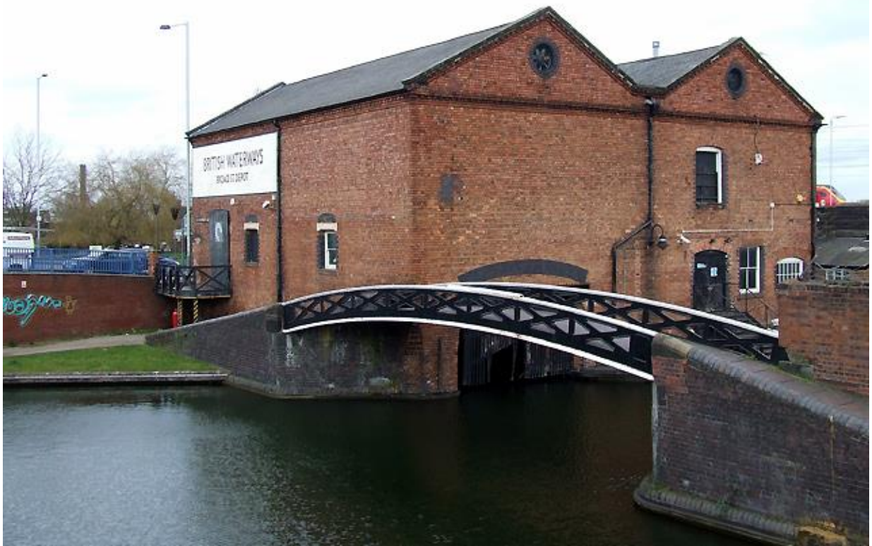
Canal Bridge Wolverhampton City Centre
